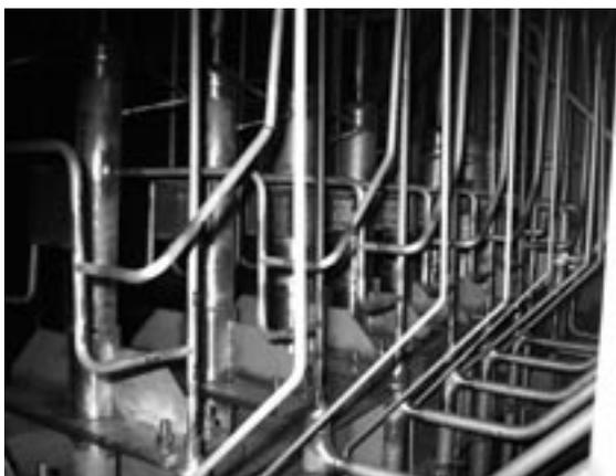
Fig. 4 Cascade connection (inside of the cold box).
