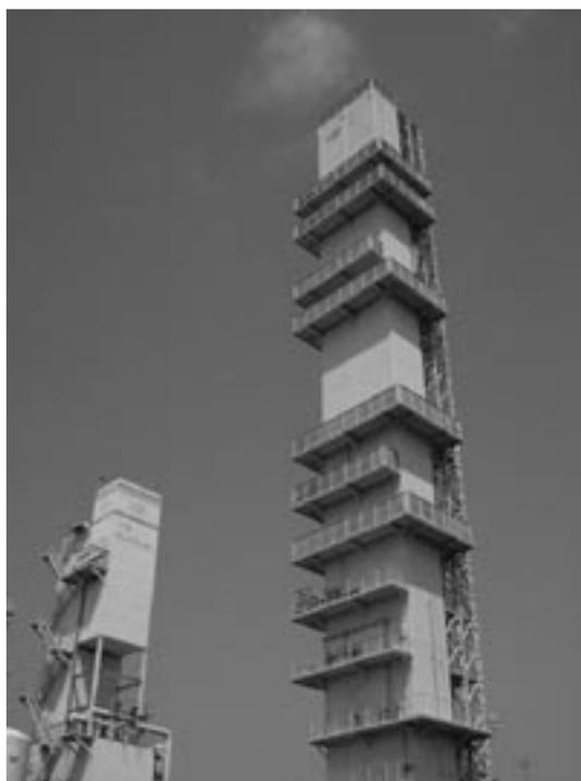
Fig. 2 Oxygen-18 separation unit (right) and existing air separation unit (left).
